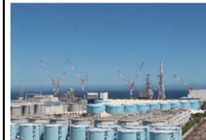
TEPCO's Fukushima Daiichi Nuclear Power Station
